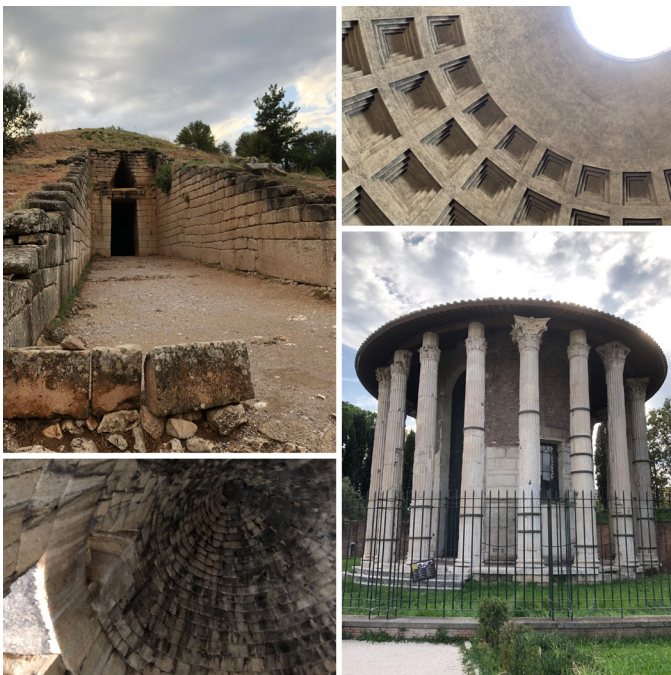
Photos by the author, clockwise from top left: Treasury of Atreus, corbelled vault of Treasury of Atreus, Temple of Hercules Victor in the Forum Boarium of Rome, concrete dome and oculus of Roman Pantheon.
